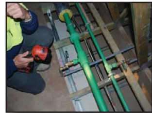
walkway in roof space
